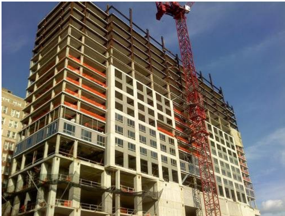
Figure 6: 360 State Street Under Construction, October 2009
