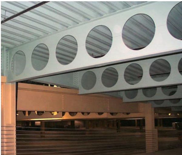
Figure 10: Cellular Beams, photo courtesy of CMC Steel Products
